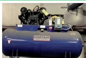
Castair Air Compressor w/ Nurse Tank
