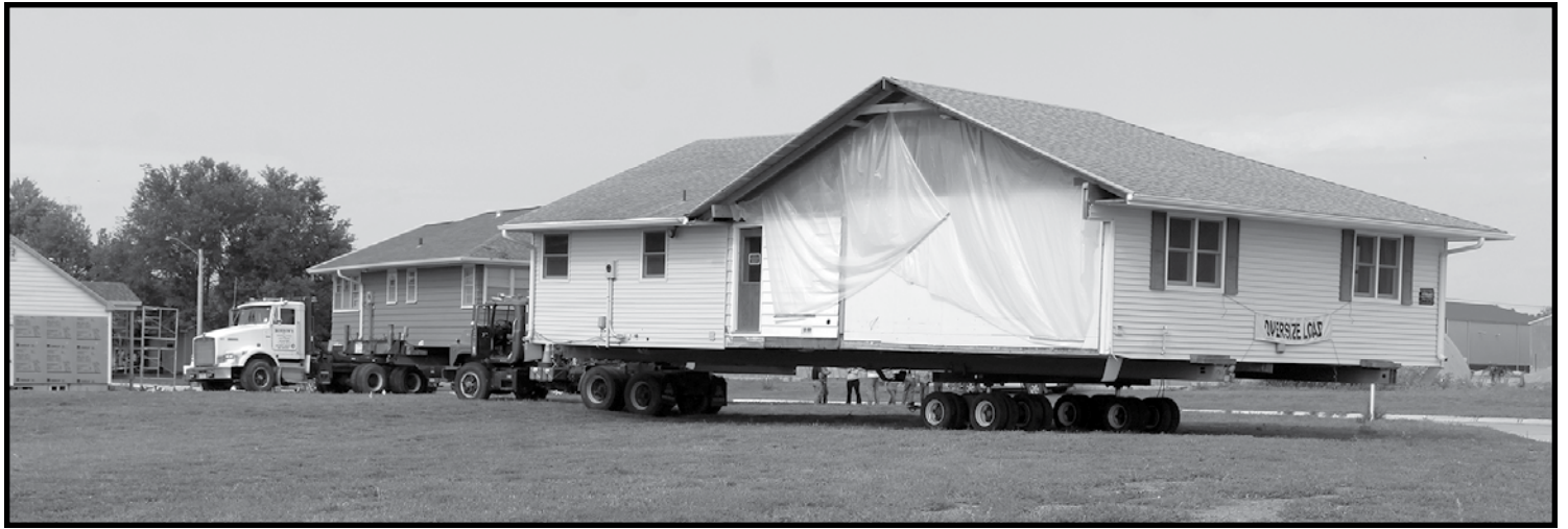
The three houses are now at their new 'home' on Chicago Street in the southwest section of Wayne. They were saved from being demolished and will soon have new owners.
