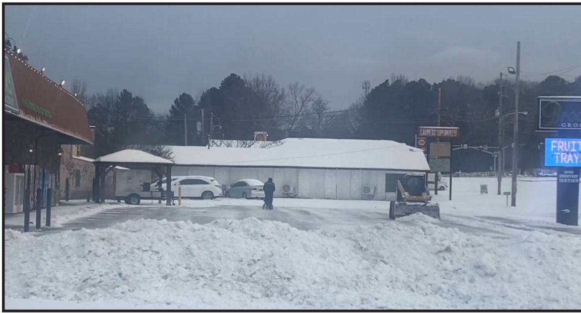
Busby Excavation Salting and Clearing the Snow & Ice at Brooks' Grocery in Iuka Before Opening Time
