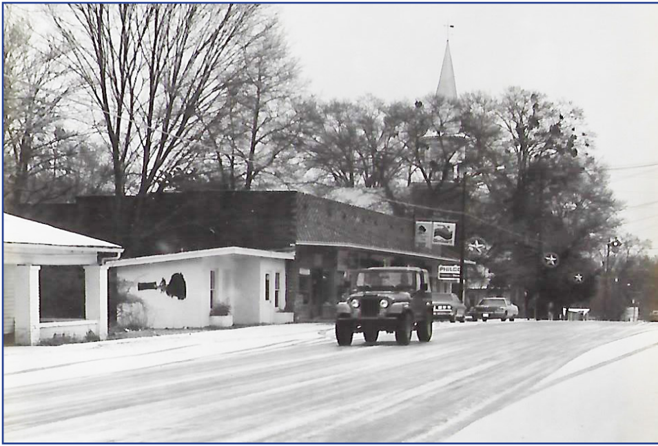
Eastport Street, maybe before the 1970's, across from Iuka Baptist Church. Building at left is now a parking lot, then there was Mr. Crossett's office and at one time this little building was the Iuka Library, then next is Strutt Edmondson's dry cleaner (Apron Museum today), The Vidette was also in this building in the 1950's. This was called the Dexter Block.
