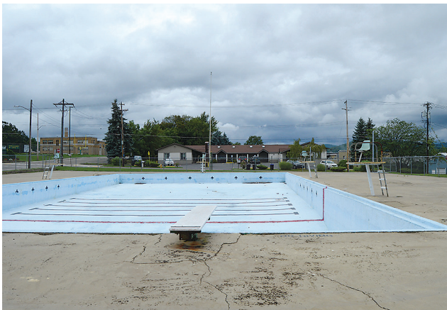
The pool before construction begins
