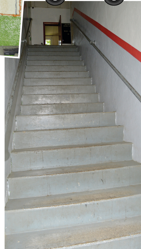
The long staircase within the current station
