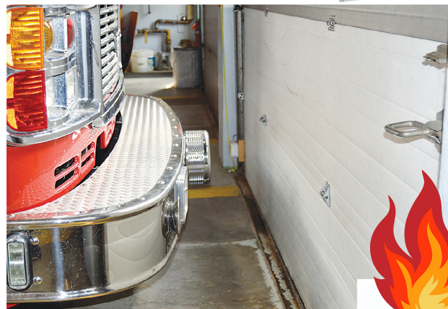
even less room between the trucks and doors on the other bay area
