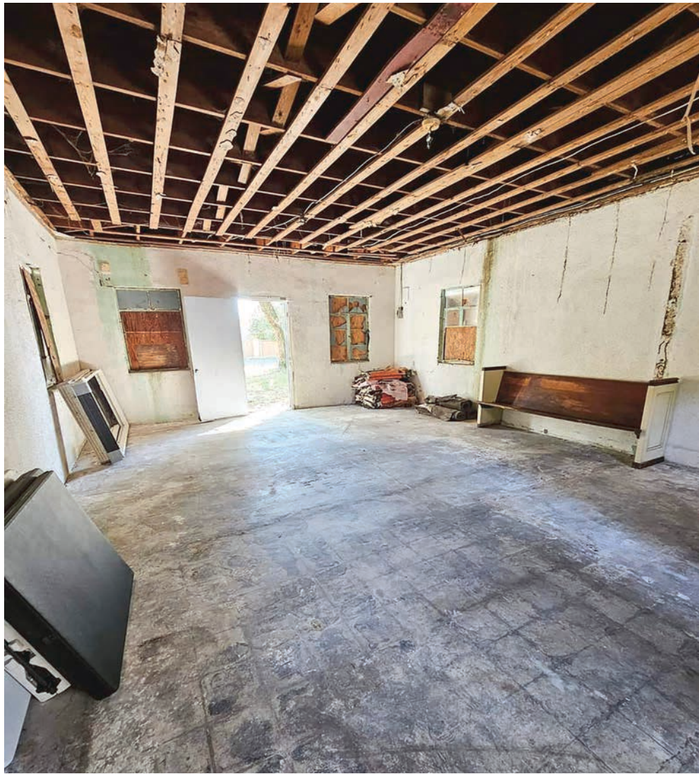
The storage unit before Gulley and her team refurbished it.
