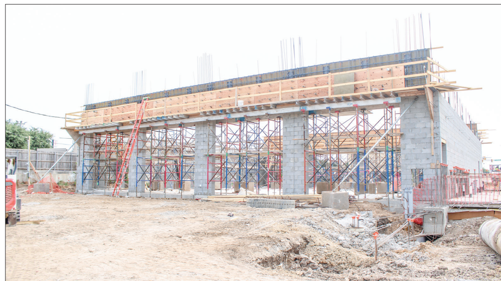
The new Lake Worth fire station being built.
