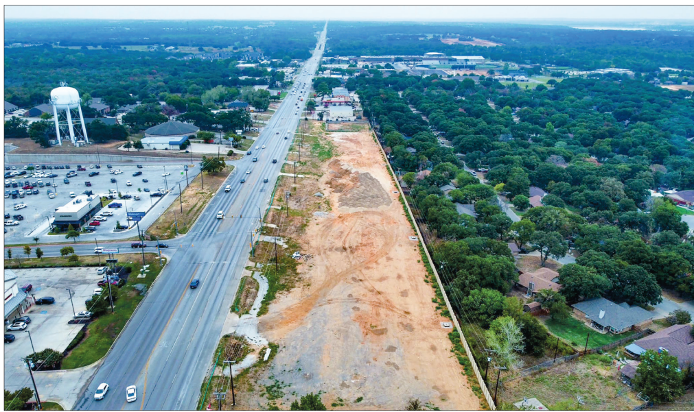
An aerial shot of the vacant property across from Walmart on Boyd Road taken via drone by part 107-certified Azle resident, Jon Lo.
