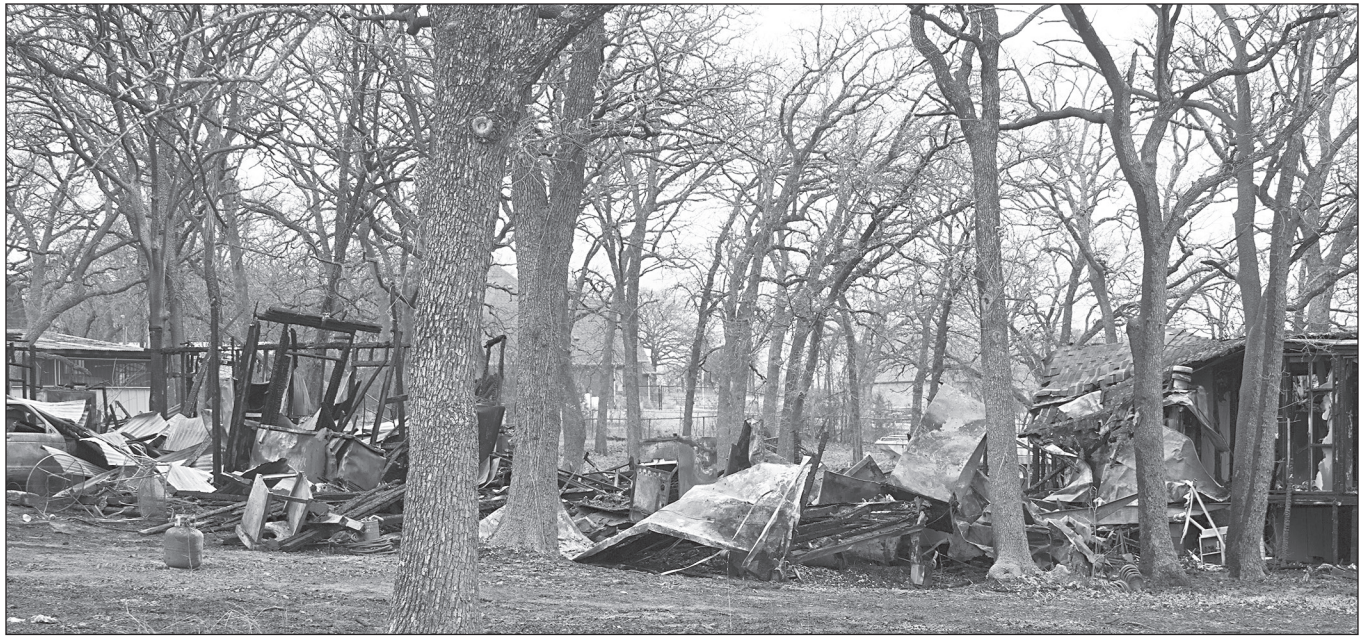
A burned-out shell is all that remains of a home in the 300 block of Turpin Drive after it was ravaged by fire Jan. 26. Photo by Carla Noah Stutsmann
