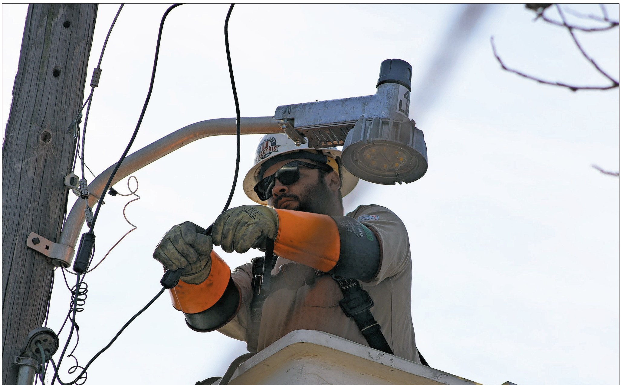
Blake Creamer, apprentice lineman, works on a line.
