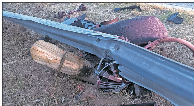
The city of Azle has spent more than $25,000 to repair guardrails damaged in accidents since last November. Courtesy photo
