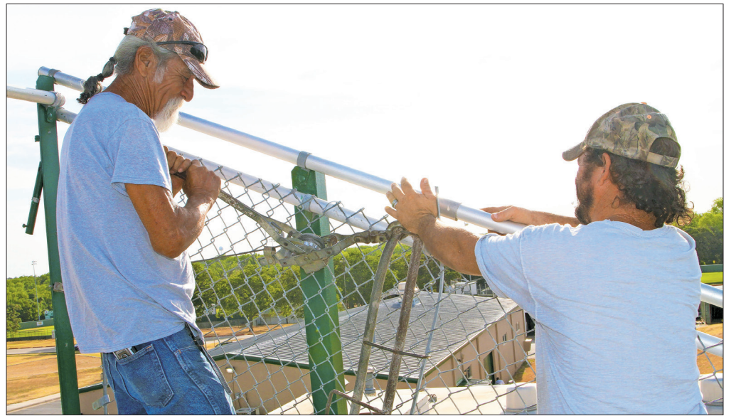
Mike Cruz and Adam Adams reattach fencing that had been removed to allow the posts to be painted.
