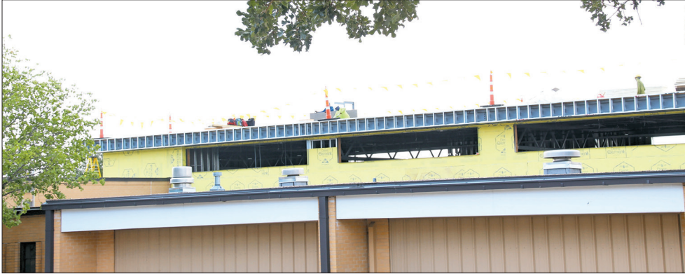
PHOTO BY JESSICA MCKINNEY New construction at Eagle Heights Elementary
