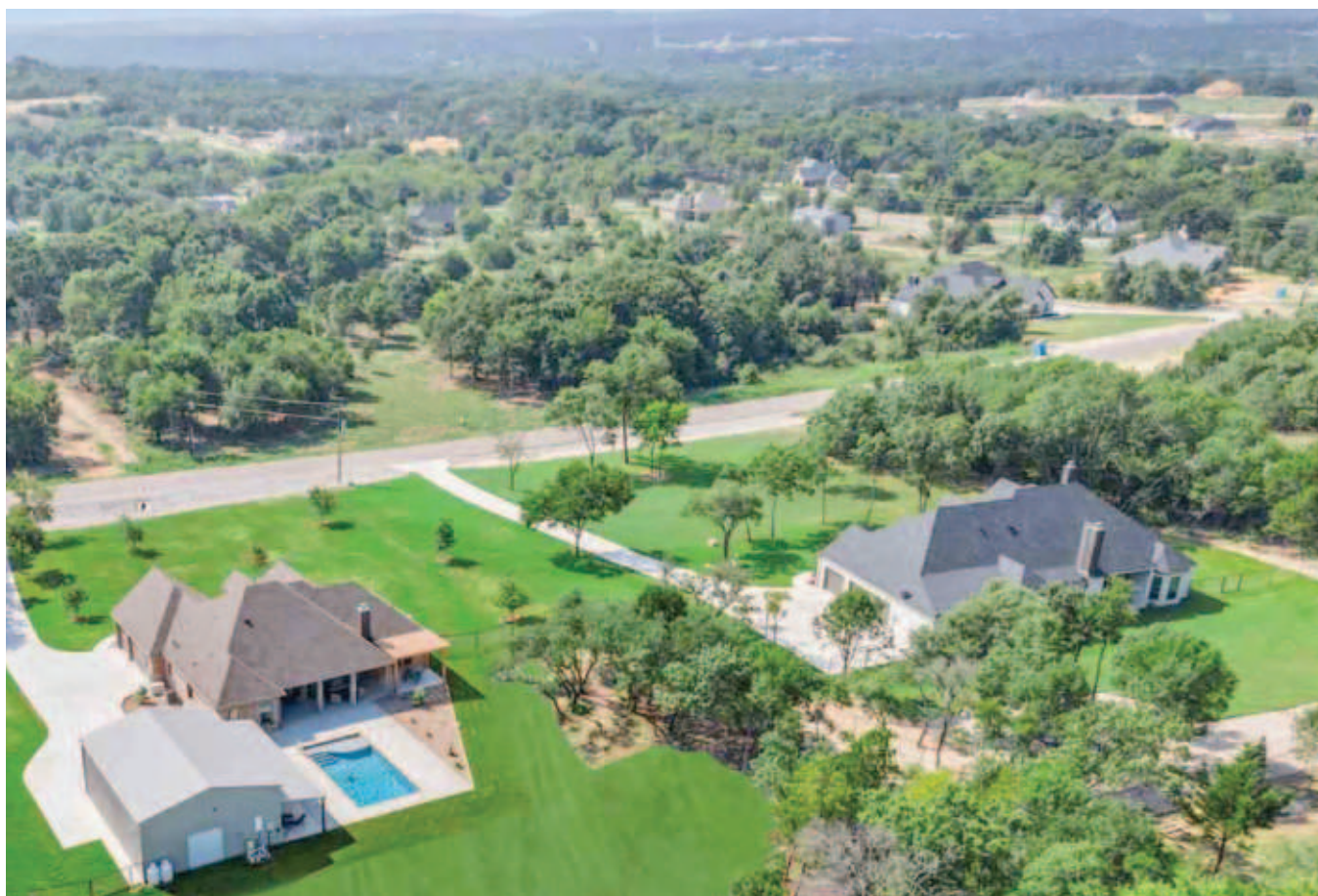
An aerial view of some of Sorrells’ custom homes.
