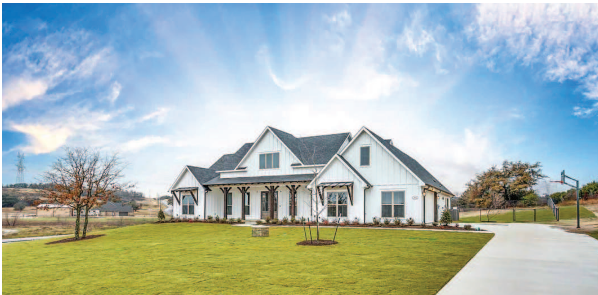
The company is very involved in the entire process of building homes and seeks to satisfy every customer.
