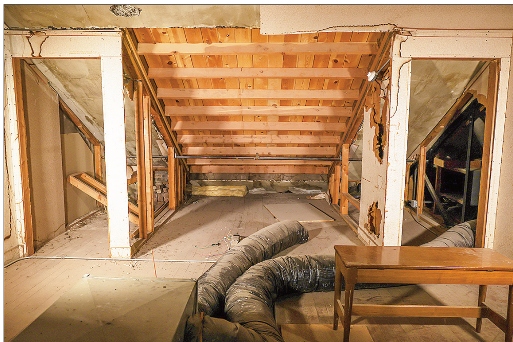
Otto Boettcher's father O. H. Boettcher donated his labor to help construct the new dormitories for returning veterans in the attic of Victory Hall. Here is a section of what remains of those dorms.
