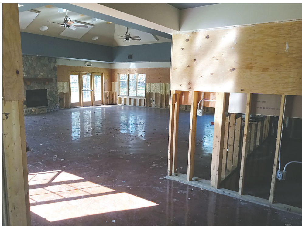
Councilperson Amy Loughlin requested the council determine whether to board the building up before temperatures begin to drop. The council agreed to seek bids for building repairs at a later date. CHRONICLE TIMES photo by CHRIS REED
