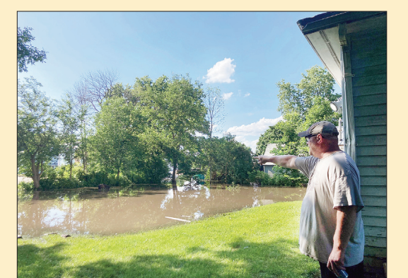
In the backyard, B.J. Habben points towards Highway 71 where the water is coming from. His garage is now skewed.
