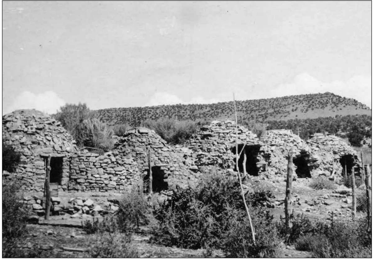
This image shows five of the six coke ovens built to provide coke for the copper mine smelters in Paradox Valley. Only one remains intact on the private Coke Oven Ranch. (Image courtesy of Rimrocker Historical Society)
