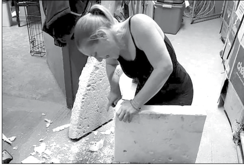
Kivi Bowersox works on tile insulation for the animal shelter.
