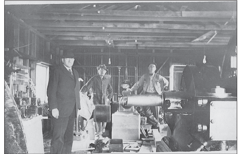
This photo, from the Standard Chemical Company collection, is a photo of Joseph Flannery of Pittsburgh, owner of the company on the left, Ray Borchardt in the center, and W. W. Gaw, superintendent of the mill on the right. They are standing with the new equipment in the power plant at the Joe Jr. Mill. (Image courtesy of Rimrocker Historical Society)
