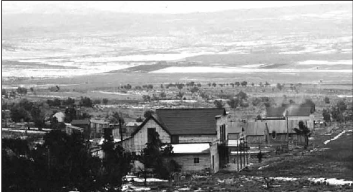
This photo shows the Vestal Hotel with the small two-room house that became the original building to hold the switchboard after it was moved from the Vestal Hotel. Both of these buildings are still standing and belong to the Dan and Cheri Cooper family. (Image courtesy of Rimrocker Historical Society)
