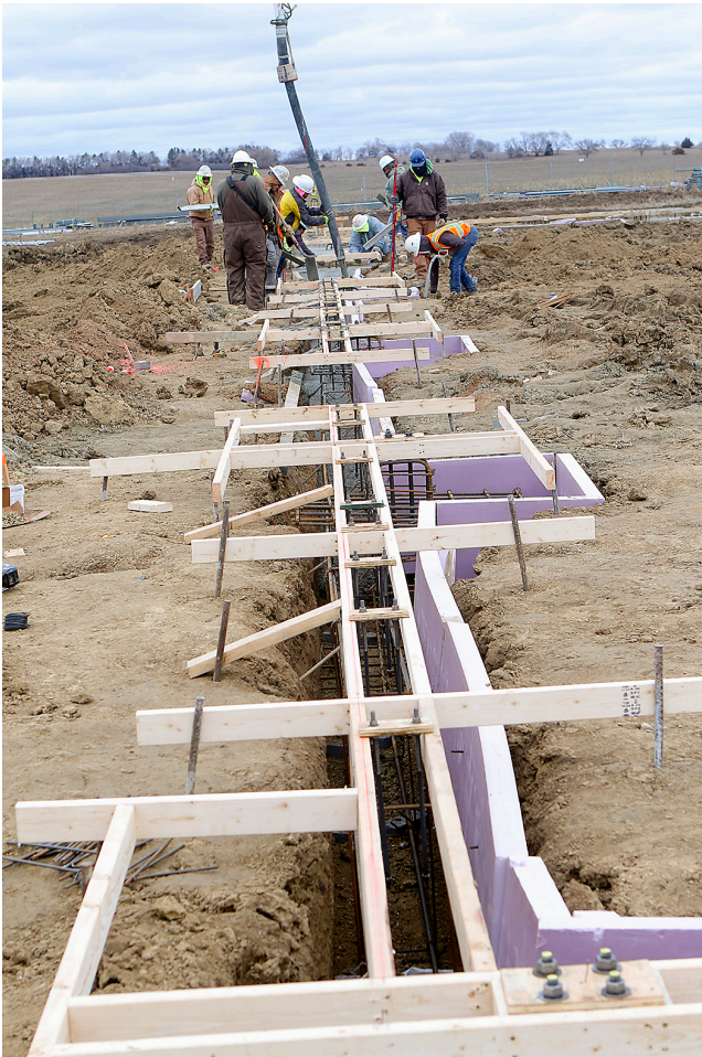
DOUG CARROLL Construction workers begin pouring the footings for the new Seward Wellness Center.
