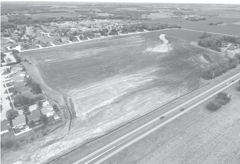
This aerial photo of the new development site east of Seward shows regrading is currently taking place for the drainage system.
