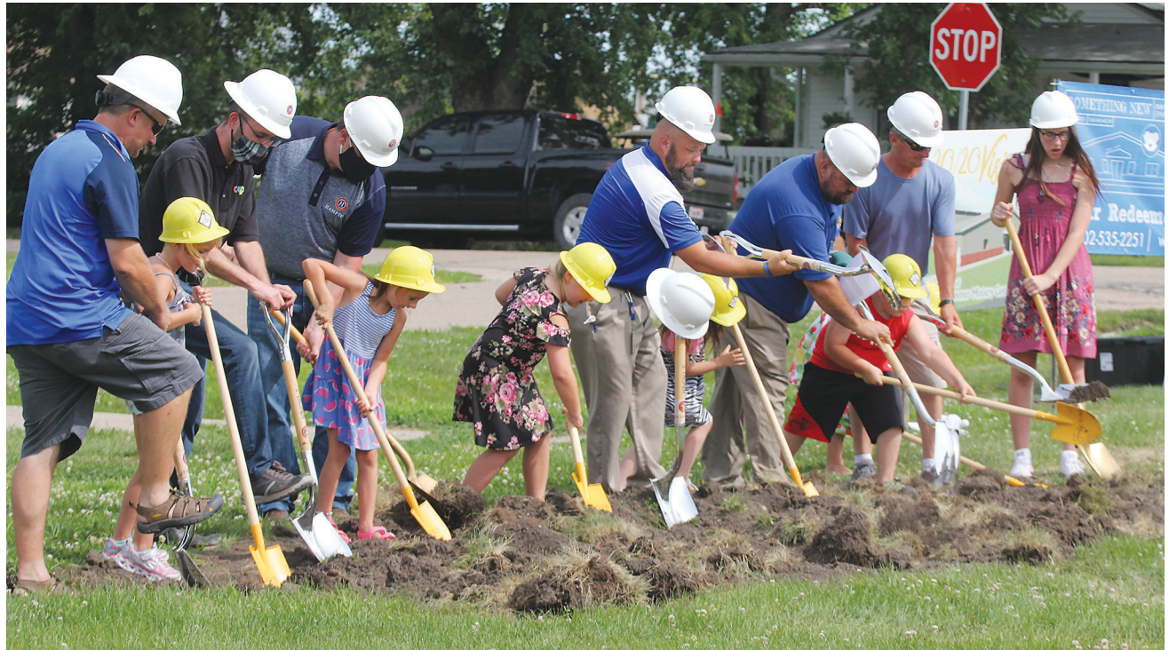
Our Redeemer Lutheran Church and School in Staplehurst broke ground July 12 for its new ministry center. Pictured wielding the shovels are, from left, Paul Duer (committee chair), Vivian Schluckebier (kindergarten graduate), Darin Blair (architect), Zoe White (kindergarten graduate), Jason Hulsebus (project manager), Saylor Wood (kindergarten graduate), Principal Harlan Anson, Aria Elmshausen (kindergarten graduate), Rev. Shawn Kitzing, Beau Alloway (kindergarten graduate), Scott Prochaska (Board of Education chair) and Mackenzie Rempel (eighth-grade graduate).
