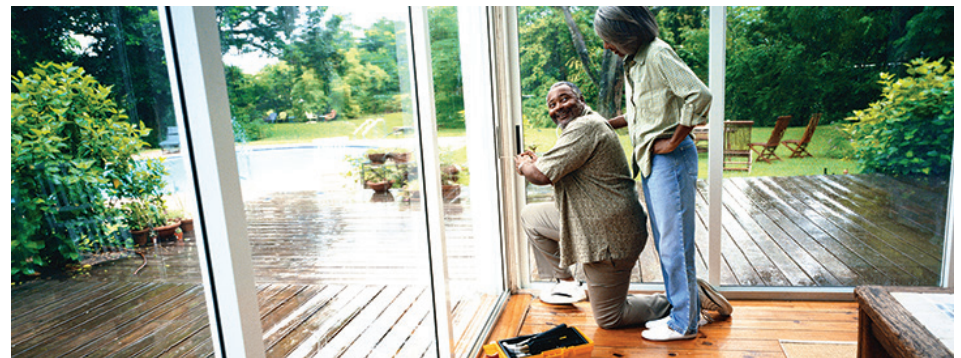
Large windows lead the pack of expected renovation trends in 2021.
