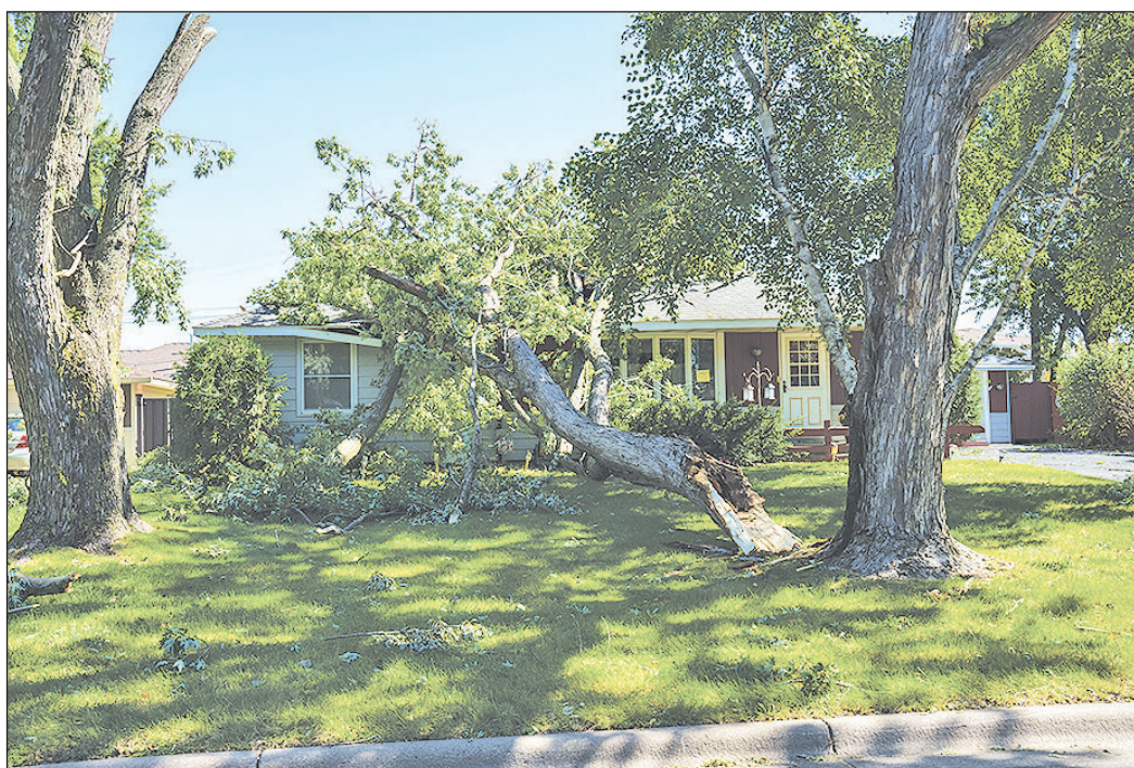
Some houses were labeled as temporarily condemned due to the size of the trees that fell on them and the damage those trees did. Owners needed to find alternative housing until the damage could be inspected and the building cleared for reentry. Photo by Bruce Karnick
