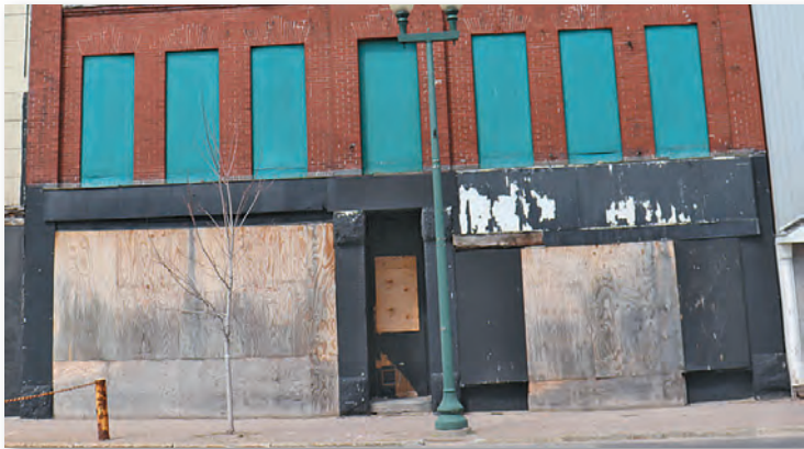
The former Massena School of Business building is slated for demolition.
