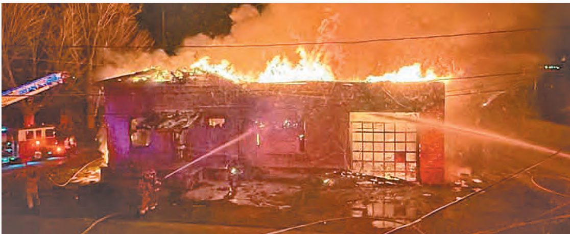
A fire at an Ogdensburg warehouse last week has raised public concerns regarding the safety of vacant buildings. Above is one of dozens of photos shared on social media by city residents.
