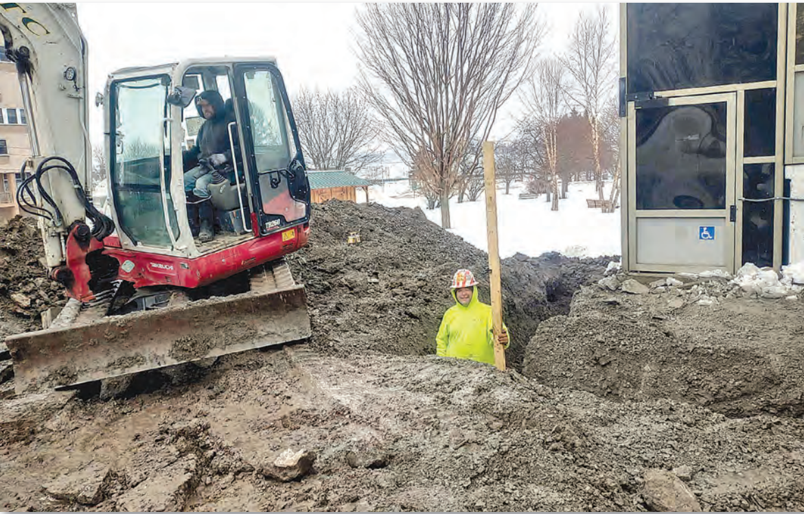
Photo courtesy of Ogdensburg Public Library The Ogdensburg Public Library has begun construction of a new lift and enclosure for access to the building.
