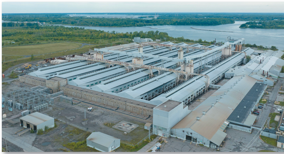
Aerial view of North Country Colocation Services in the former Reynolds/Alcoa plant, Massena.
