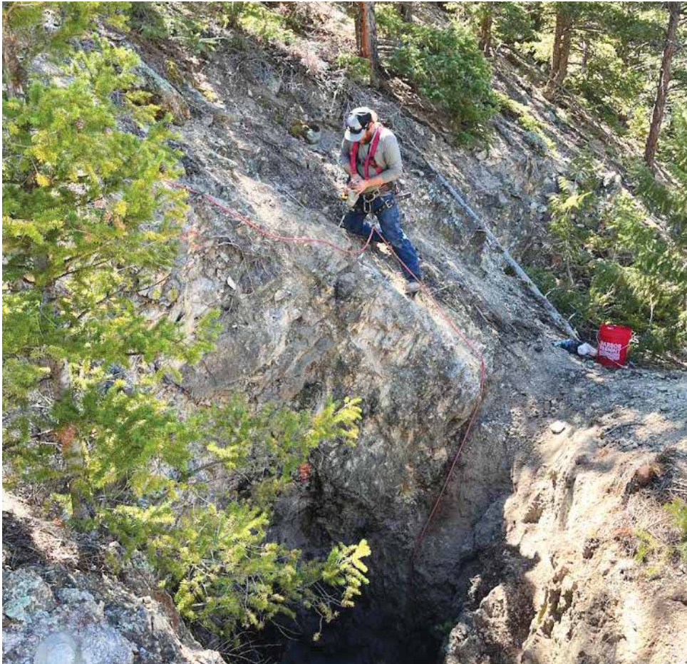
Equipment must be hauled in Left: Preparing a shaft for a cable net closure by drilling anchor bolts into the stable rock around the side of the mine opening. Right: Pack animals are the only way to get to some of the remote mines.
