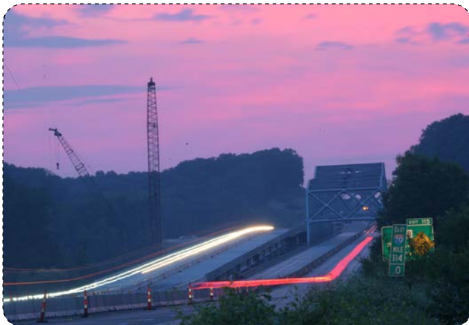
Kate Cassady with the Columbia Missourian took first with this Best Feature Photograph capturing the old I-70 bridge spanning the Missouri River weeks before its planned demolition.
