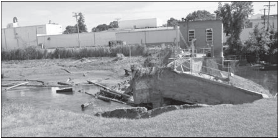
Dwight Shanak, operator of the powerhouse on the Manawa dam, explained to the city that the dam was timber crib dam, built similar to a log cabin and filled with rock and concrete. An underflow formed underneath the dam and Shanak said the dam's lifespan ran out 50 years ago. Emily Doud Photo
