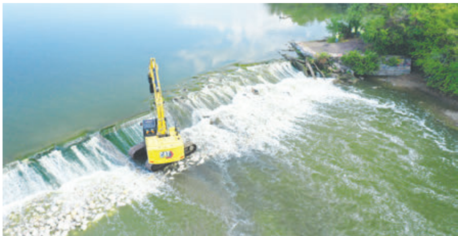
September 20, 2024, work begins on the removal of the Carpentersville dam, scraping/chiseling off one foot of the approximately 4 to 6-foot thick, 8-foot high aging structure one day at a time. Notice the vibrancy of the water, the sandy shores and bottom, downstream from the dam versus the silt-trapping, low-oxygen "dead zone" stillness of water behind the dam.
