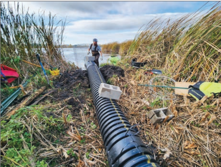
Dan Fuhs, co-owner of Native Range Ecological, installs a pond leveler in October 2023, near the village of Rio.
