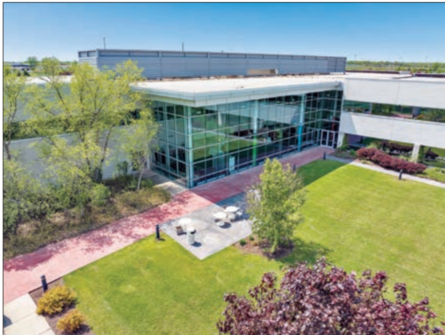
Park Place Holdings, a De Pere-based commercial real estate investment firm, recently acquired the office facility at 3500 Packerland Dr., Ashwaubenon. Submitted photo
