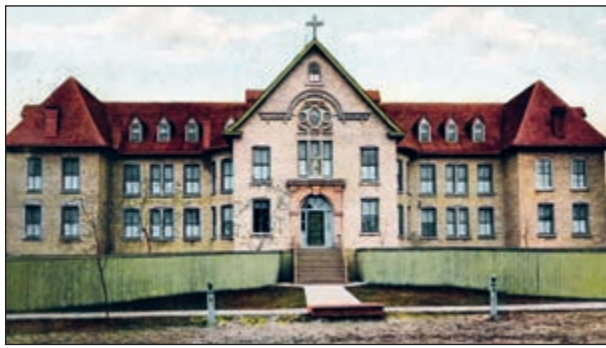
In 1896, the sisters sold the three-lot property facing St. John’s Park to the Sisters of St. Joseph, as their new convent was being completed on Webster Avenue and Porlier Street across from St. Vincent’s Hospital.
