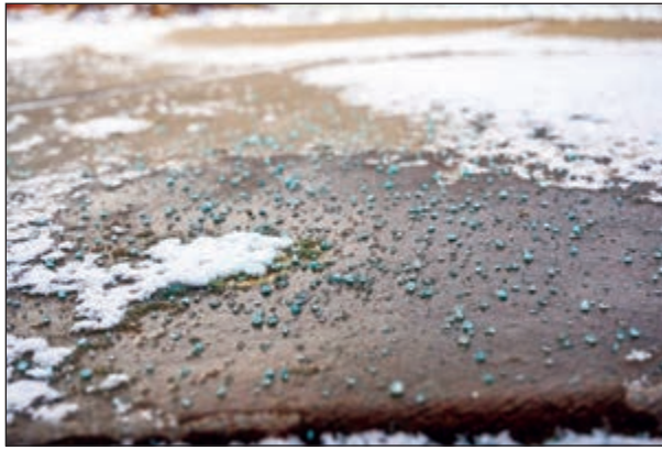
Over-salting can lead to chloride buildup in lakes, streams and groundwater. Stock Photo
