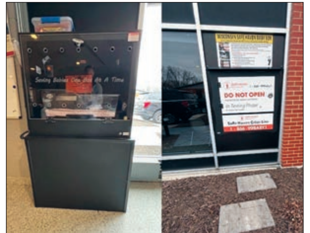
The exterior door locks automatically when a newborn is placed inside, and an interior door allows medical personnel to promptly and securely retrieve the baby, ensuring immediate care and protection. Submitted photo
