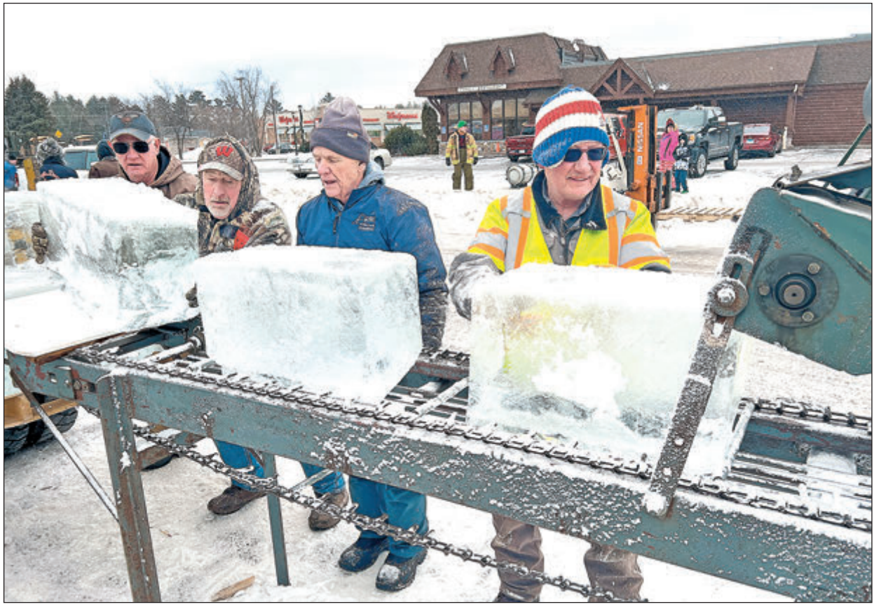
Former Eagle River Fire Department Fire Chief Pat Weber (right) and volunteers guided 13-inch blocks of crystal clear ice through a shaver to make them a uniform size prior to construction of the Eagle River Ice Castle near the railroad depot.
