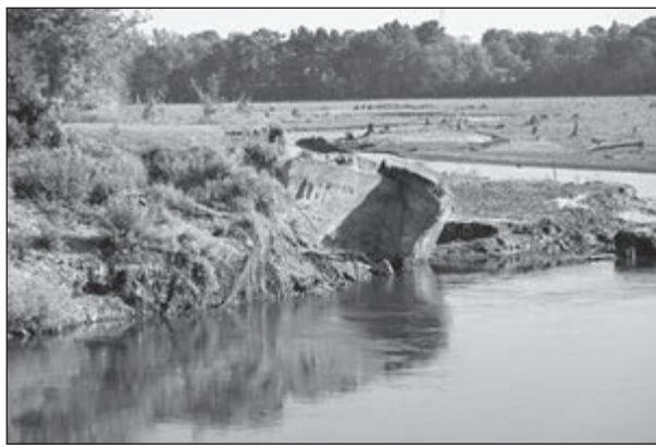
The shore on the Sturm Memorial Public Library is continuing to erode and will need to be stabilized before any potential spring run-off. Emily Conroy Photo
