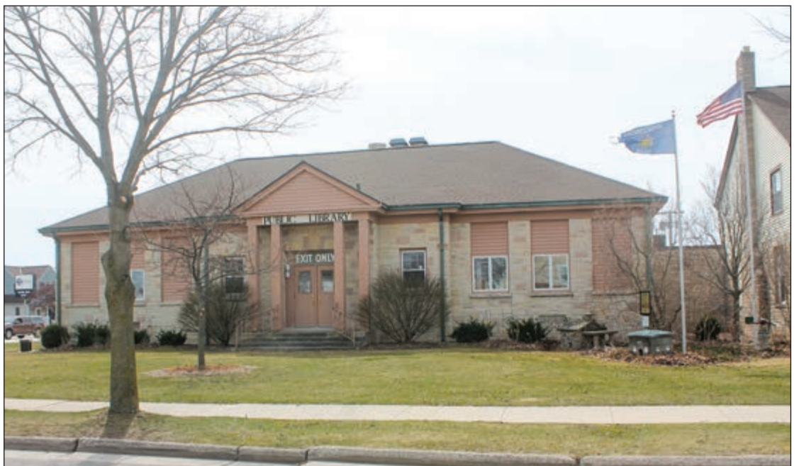
Potential sites for the project included Fremont Street where the city hall and library are located, property at Sunset Avenue and Rabas Street and a site at Sunset and Feld Street. File photo
