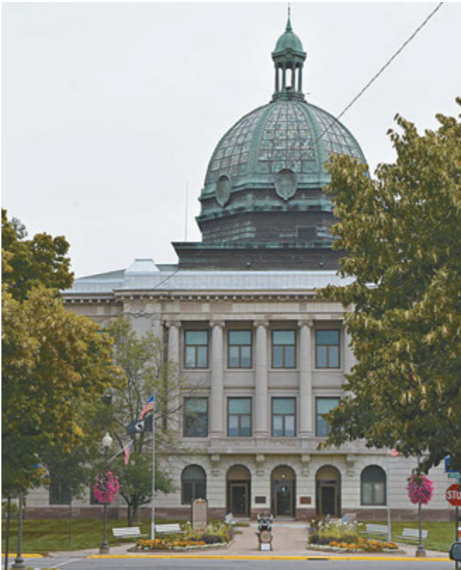
The historic Oneida County Courthouse in downtown Rhinelander. MMC photo
