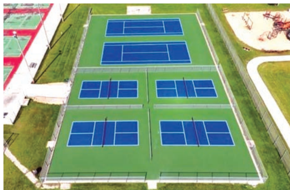
An aerial view of the OSMS Court Complex at Higley Field, with two finished tennis courts and four new pickleball courts.
