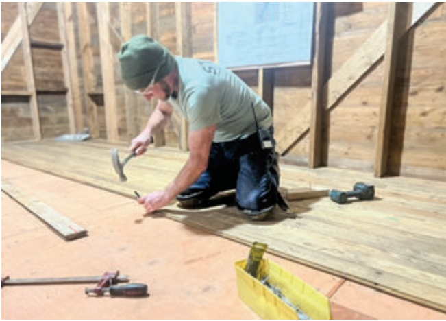
David Haack installs the original flooring. The house was disassembled and transported to Heritage Hill in 18 pieces, including 12 wall sections, four roof sections and two floor sections, where it is being reassembled and prepared for an early May opening.
