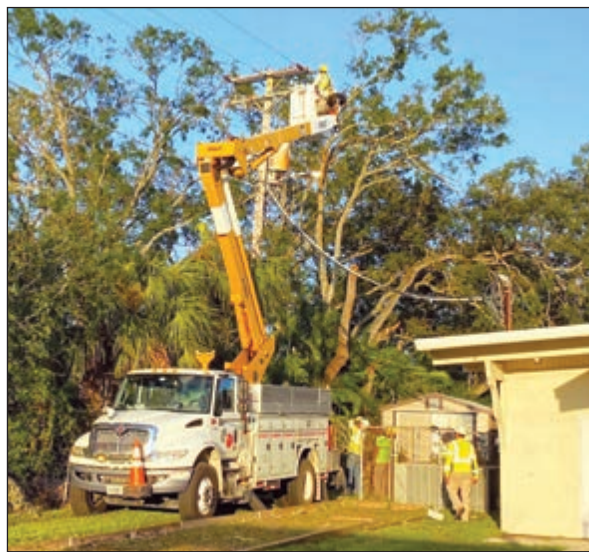
A WPS crew works to restore a power line in Florida.
