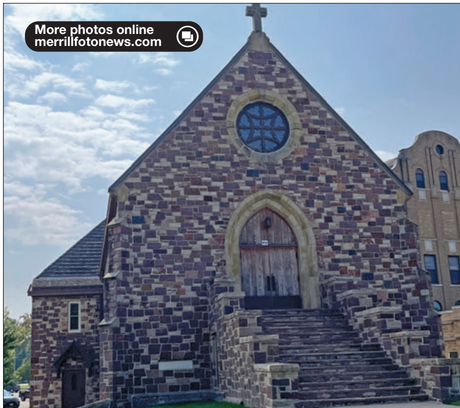
The Holy Cross Chapel sits high on Holy Hill, attached to Aspirus Merrill Hospital. The building is set for demolition later this month to make way for hospital expansion. Tina L. Scott photo.
