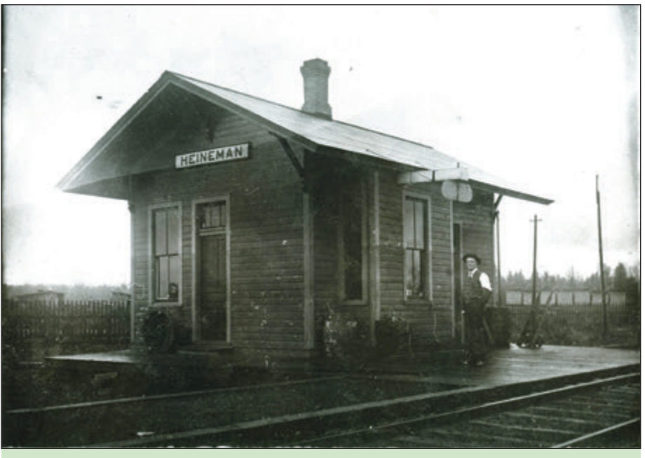
The Heineman Depot. Photos courtesy of Tom Burg.
