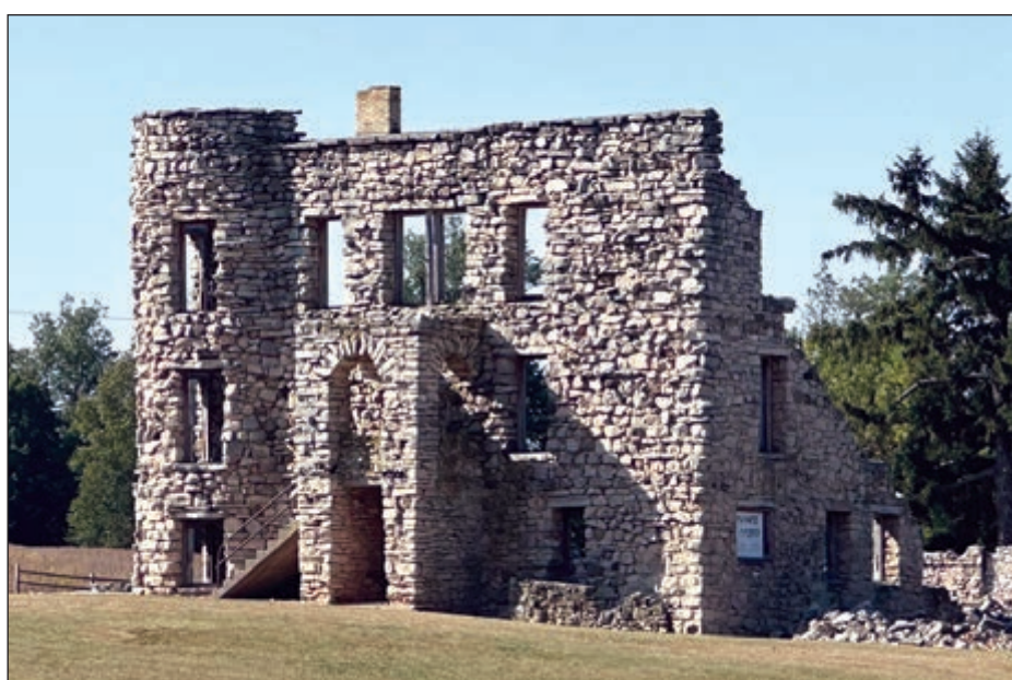
The ruins of the Maribel Caves hotel, built by Austrian immigrant Charles Steinbrecker in 1900. Kris Leonhardt photos
