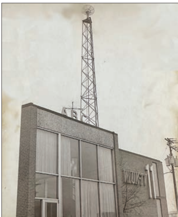
Hutchison said that by the time Post went to get money for the WLUK building, the company was cash poor but somehow managed to borrow $300,000 to complete the building. WLUK photo
