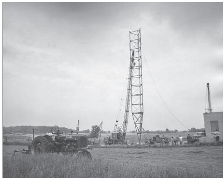
The transmission tower under construction north of Oconto.
