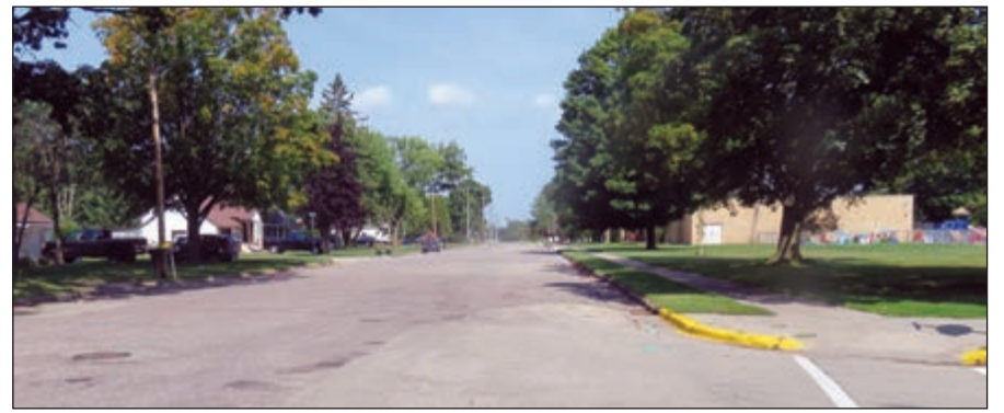
Clintonville received a Community Development Block Grant Public Facility grant to help fund reconstruction of Harriet Street and underground utilities, including water, wastewater and storm sewer. Bert Lehman Photo
