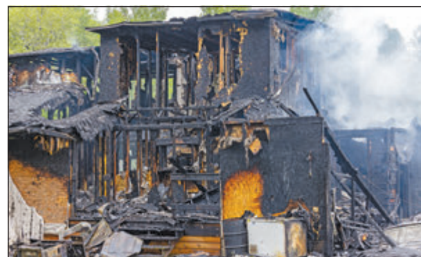
A house fire in the Town of Rock Falls completely destroyed the home. Joseph Frederick photo.
